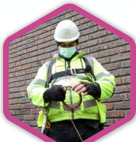
Workers will connect 14,000 council homes by 2023
