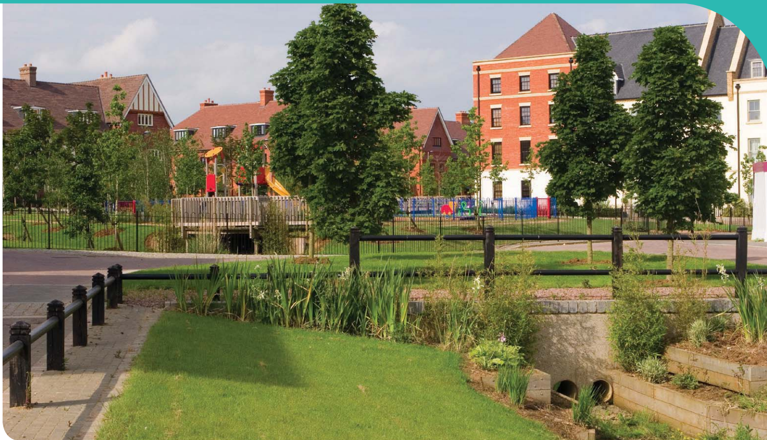
Recent high quality, sustainable, suburban development: an example from Upton, Northampton.
