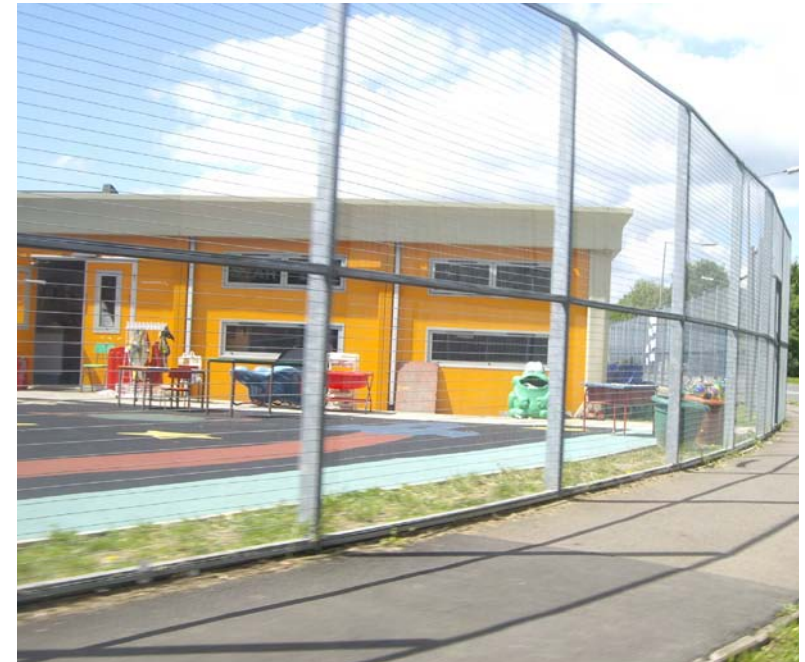
Primary School, Lanacre Avenue
