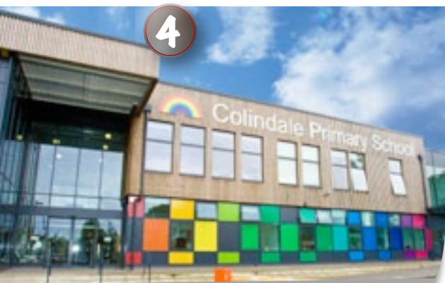
Colindale, the borough's newest primary school building: opened in spring 2012
