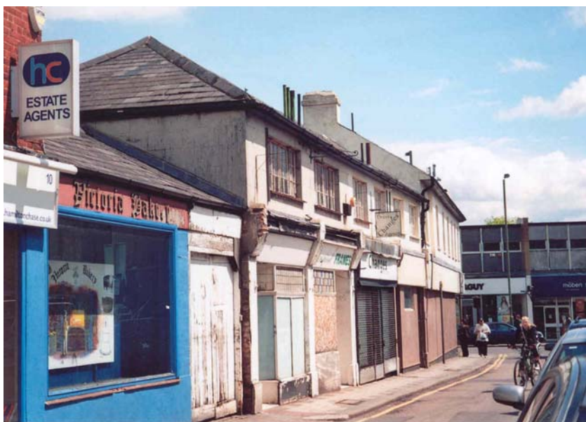
Nos. 2 to 8 Union Street (derelict shops)
