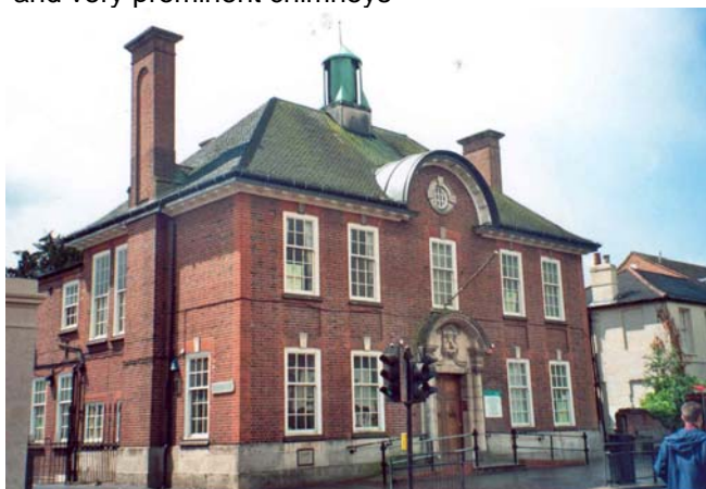
Former Registry Office, no. 29 Wood Street (recently Grade II listed)
