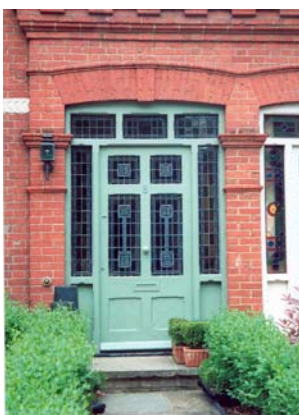
Door at no. 8 Ravenscroft Park
