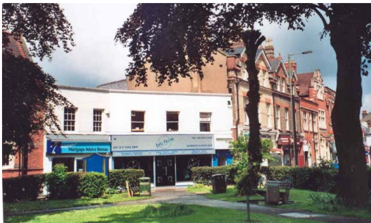
North West views onto High Street
