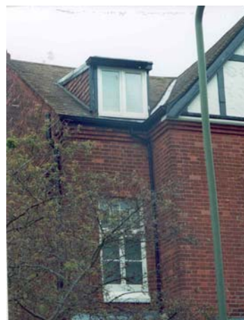
Dormer window at no. 12 Ravenscroft Park
