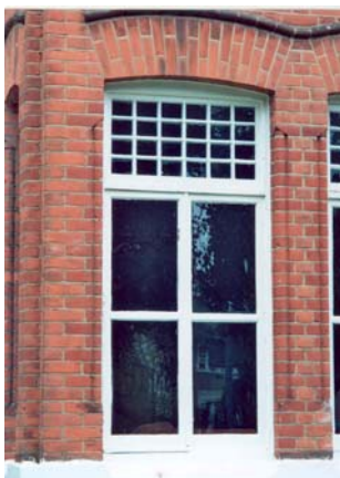
Unusual window design at no. 15 Ravenscroft Park
