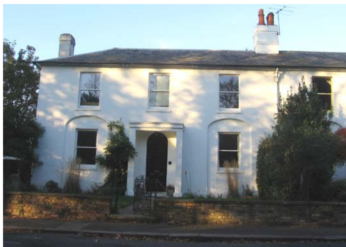
Grimsdyke, The Avenue
