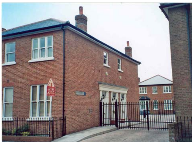
Recent gated development (Leinster Mews) Union Street
