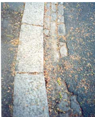
Evidence of historical cobbles, Ravenscroft Park
