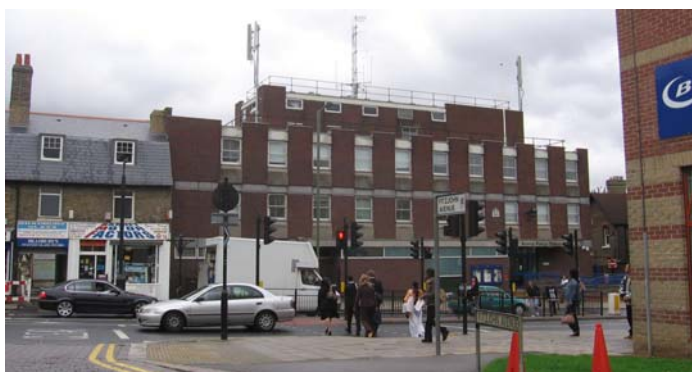
Police Station, High Street
