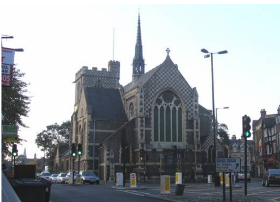
The eastern elevation of St John the Baptist Church
