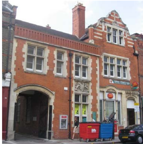
Post office, 63 High Street
