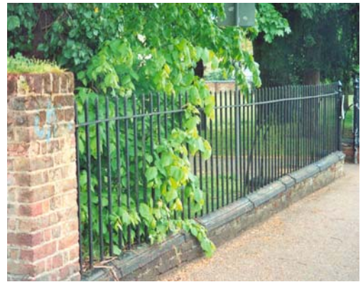
Railings surrounding Ravenscroft Park
