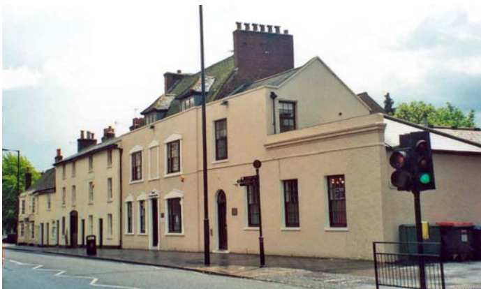
Nos.15 to 27 Wood Street
