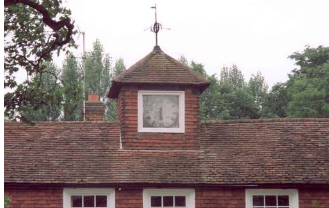
Clay roof tiles on Grange House in Grange Avenue
