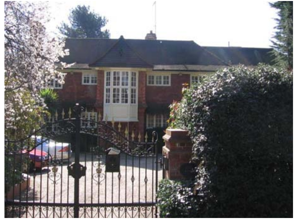
East Ridge, no. 137 Totteridge Lane
