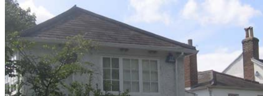
Welsh slate roof at Southerhay, Totteridge Village
