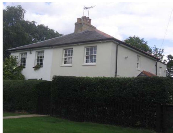
Beaconsfield Cottages, Totteridge
