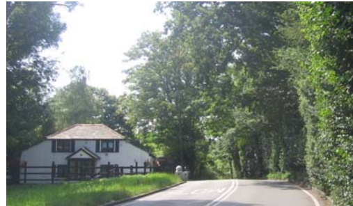
Looking east along Totteridge Common , Damson Cottage (no. 59 Totteridge Common)
