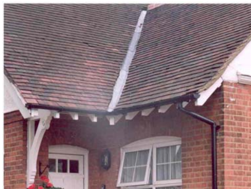
Over-sailing eaves with exposed rafter feet
