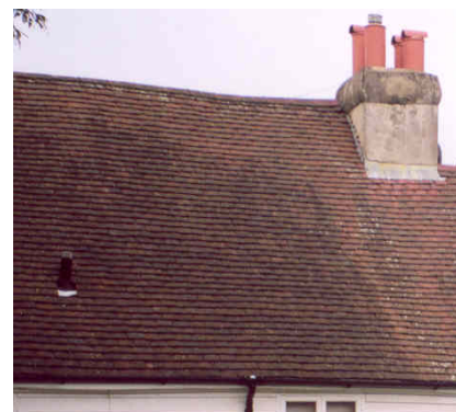
Undulating red and brown clay tiled roof at Rosebank Cottage
