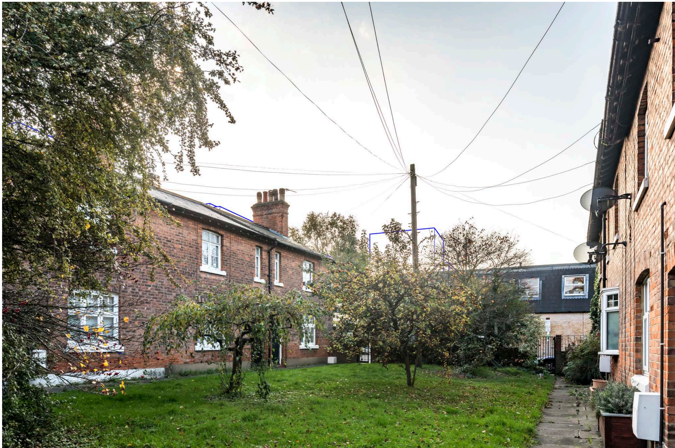
Right Application Scheme (November 2022) showing Cumulative Schemes 1-13 Cricklewood Lane (18/6353/FUL) and 194-196 Cricklewood Broadway (17/0233/FUL) (19/5339/NMA)
