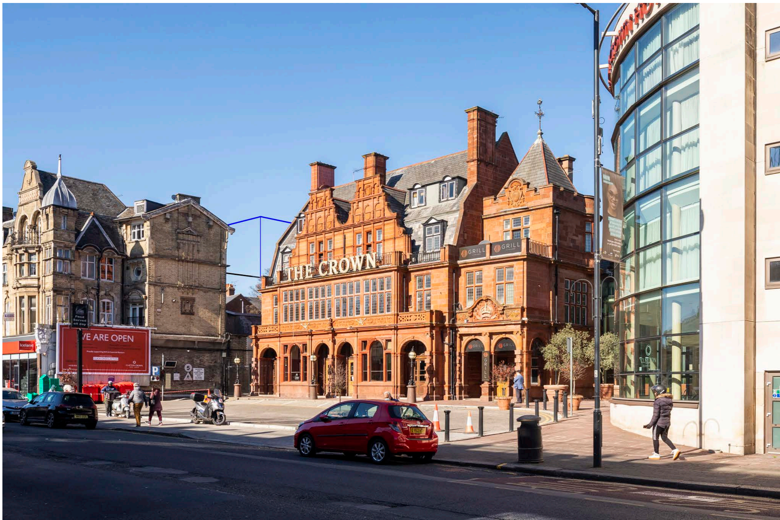
Right Application Scheme (November 2022) showing Cumulative Schemes 1-13 Cricklewood Lane (18/6353/FUL) and 194-196 Cricklewood Broadway (17/0233/FUL) (19/5339/NMA)
