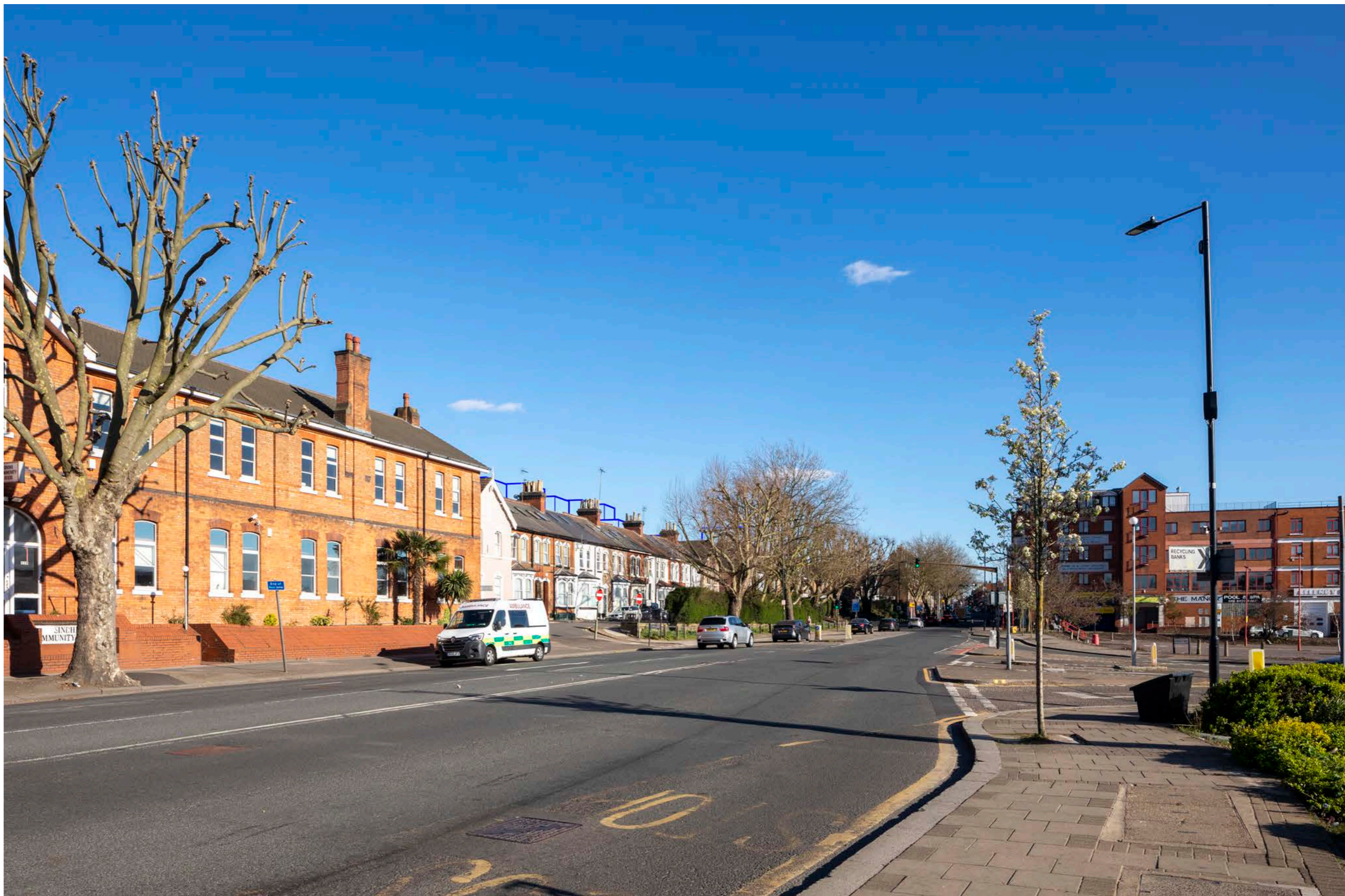
Right Application Scheme (November 2022) showing Culmulative Schemes 1-13 Cricklewood Lane (18/6353/FUL) and 194-196 Cricklewood Broadway (17/0233/FUL) (19/5339/NMA)
