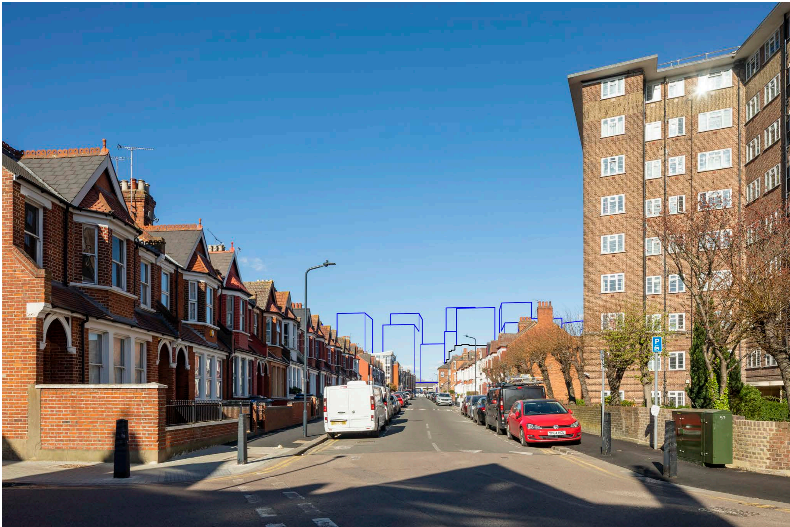
Right Application Scheme (November 2022) showing Cumulative Schemes 1-13 Cricklewood Lane (18/6353/FUL) and 194-196 Cricklewood Broadway (17/0233/FUL) (19/5339/NMA)
