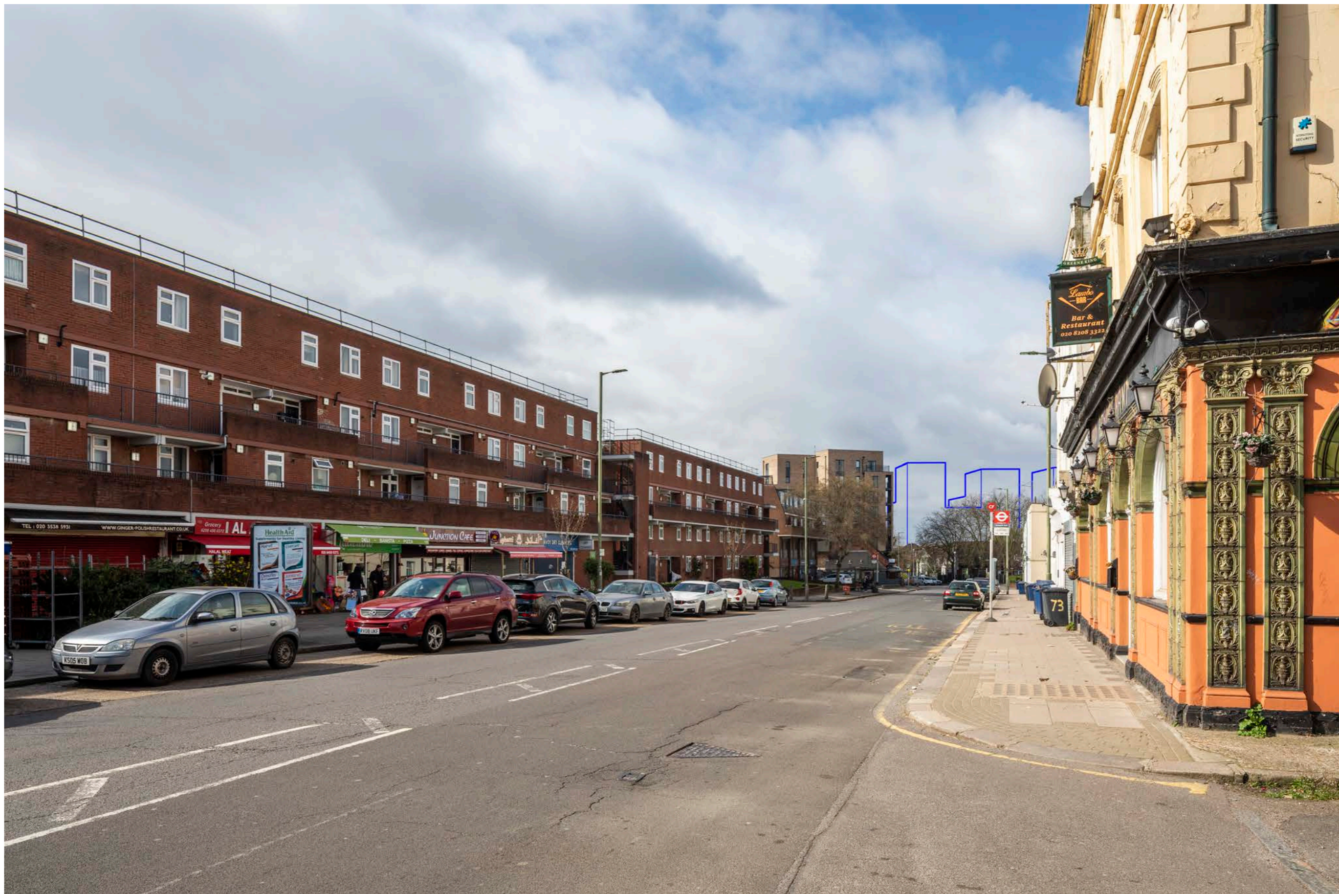
Right Application Scheme (November 2022) showing Culmulative Schemes 1-13 Cricklewood Lane (18/6353/FUL) and 194-196 Cricklewood Broadway (17/0233/FUL) (19/5339/NMA)
