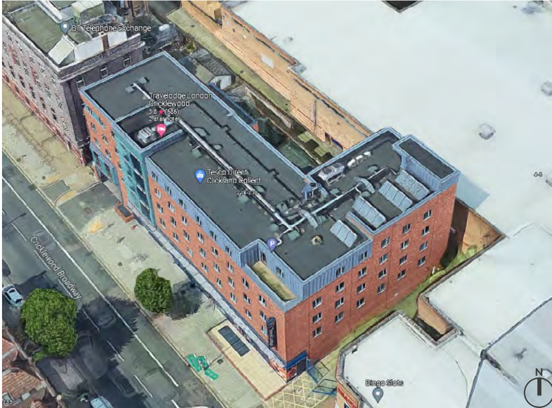
Fig. 16: Existing PV Panels - Aerial view
