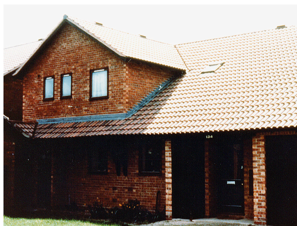
Figure 36: In these passive solar homes, a variety of front door positions and a mixture of garages and car ports produce attractive north façades
