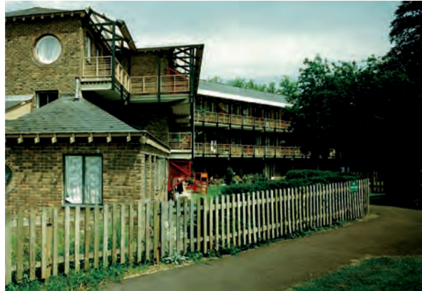
Figure 24: In this housing association scheme, solar shading is provided by balconies and overhangs
