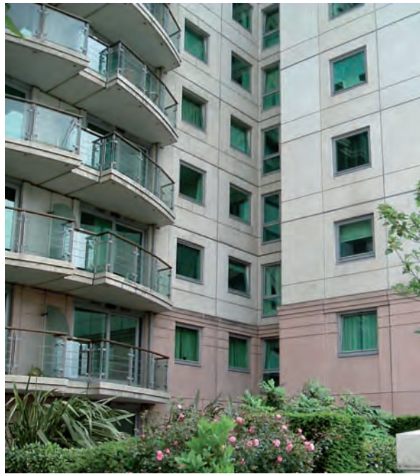
Figure 6: Windows near internal corners, such as the corners of courtyards, are usually heavily obstructed
