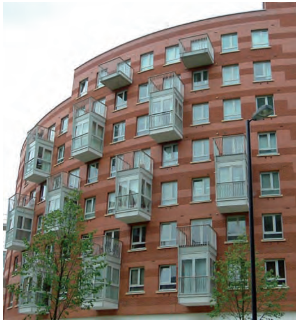
Figure 13: This North London development (architects CZWG) has staggered balconies to minimise obstruction to living rooms. Where a balcony is above a living room the obstructed area has been modified to form an unobstructed bay window.
