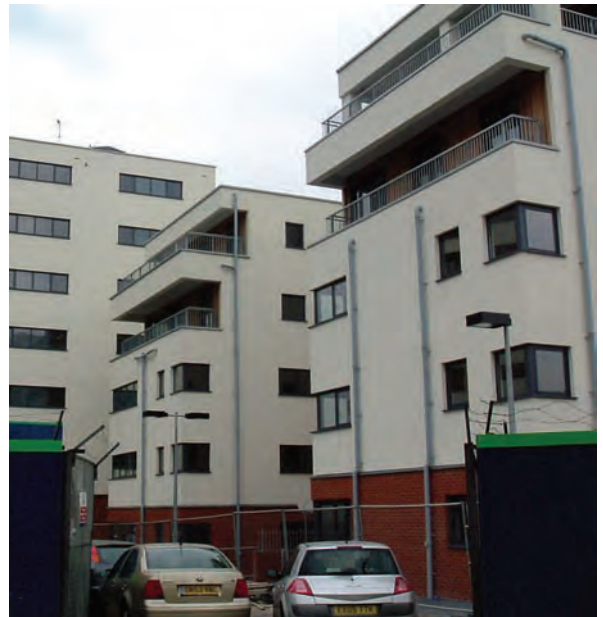
Figure 8: A white finish to external walls, as in this North London development (architects Sheppard Robson), can increase reflected light. However, windows will tend to reduce the overall effective reflectance.
