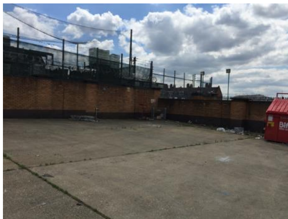
Plate 4 Service Yard (TN3) Area with ephemeral vegetation
