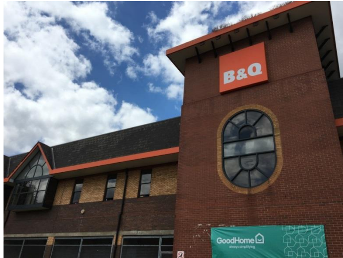
Photograph 1 Building 1 (Southern elevation)
