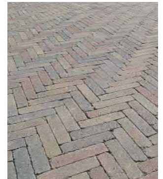
✗ Non-stretcher-bond patterns on main footways and carriageway not permitted
