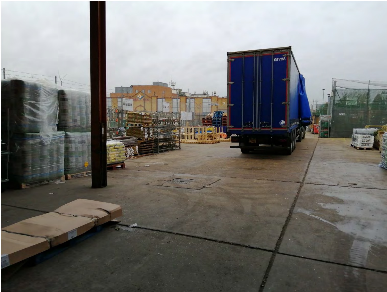
Plate 5 West facing view of the B&Q delivery and stocking yard accessed from Depot Approach road
