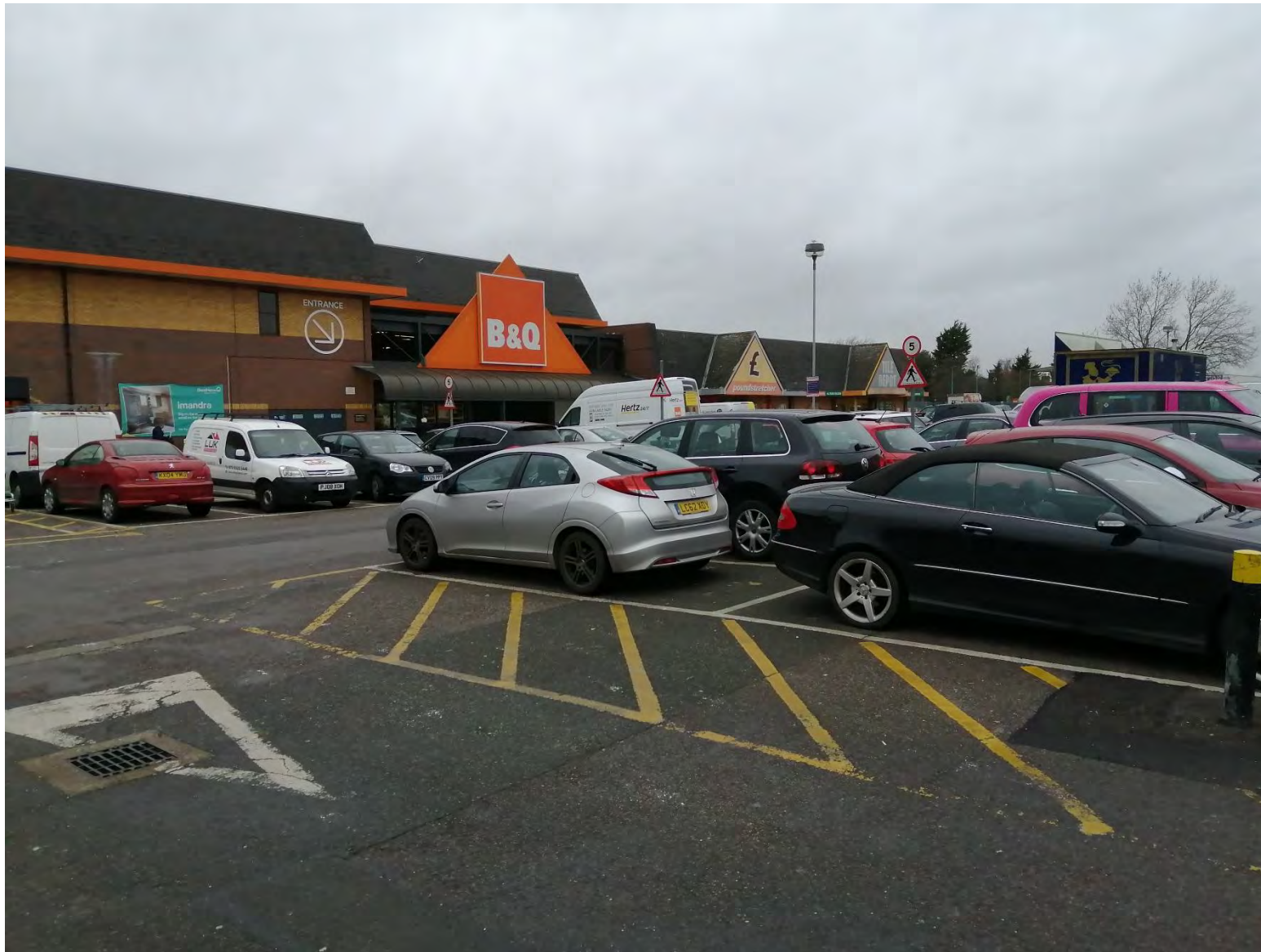
Plate 2 West facing view of the commercial properties present on Site viewed from the western boundary
