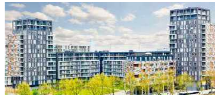
Montreaux, Indecon Court, Tower Hamlets
