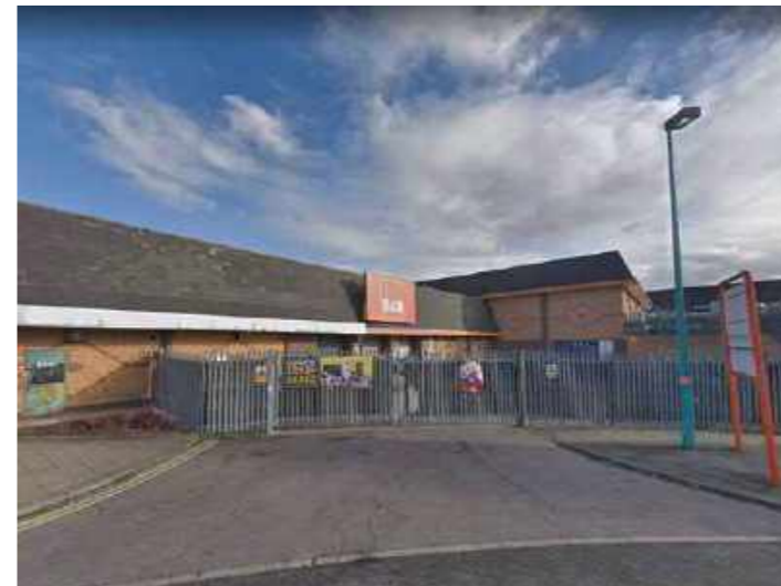
Existing service vehicle access from Depot Approach
