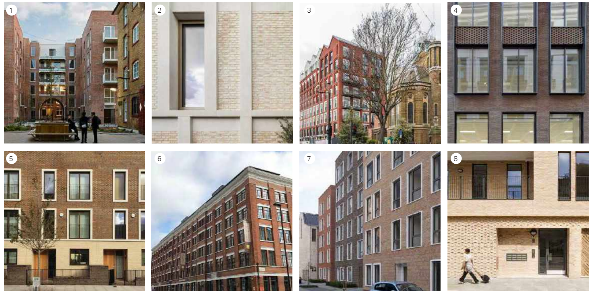
Contemporary and appropriate interpretations and expressions of the existing materiality and architectural features of the surrounding context
