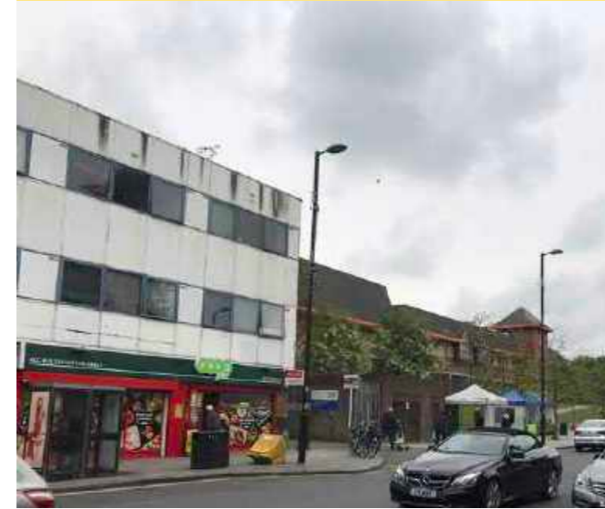
Repair existing Cricklewood Lane commercial frontage
