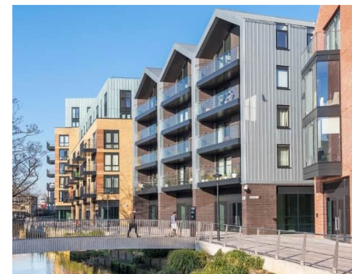
Figure 3.4 EPR Architects, The Ram Quarter, Wandsworth
