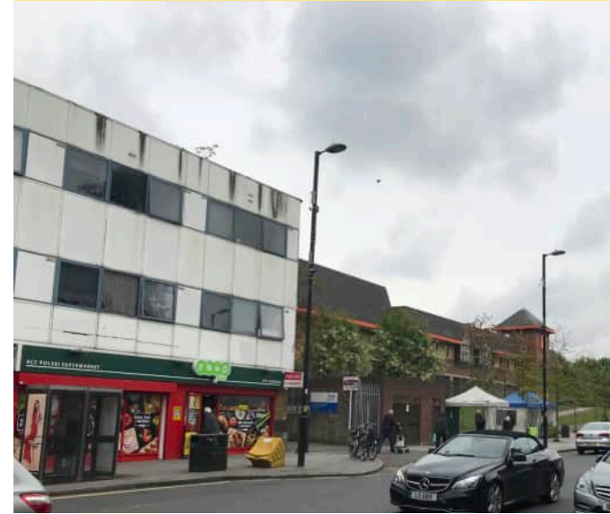
Repair existing Cricklewood Lane commercial frontage
