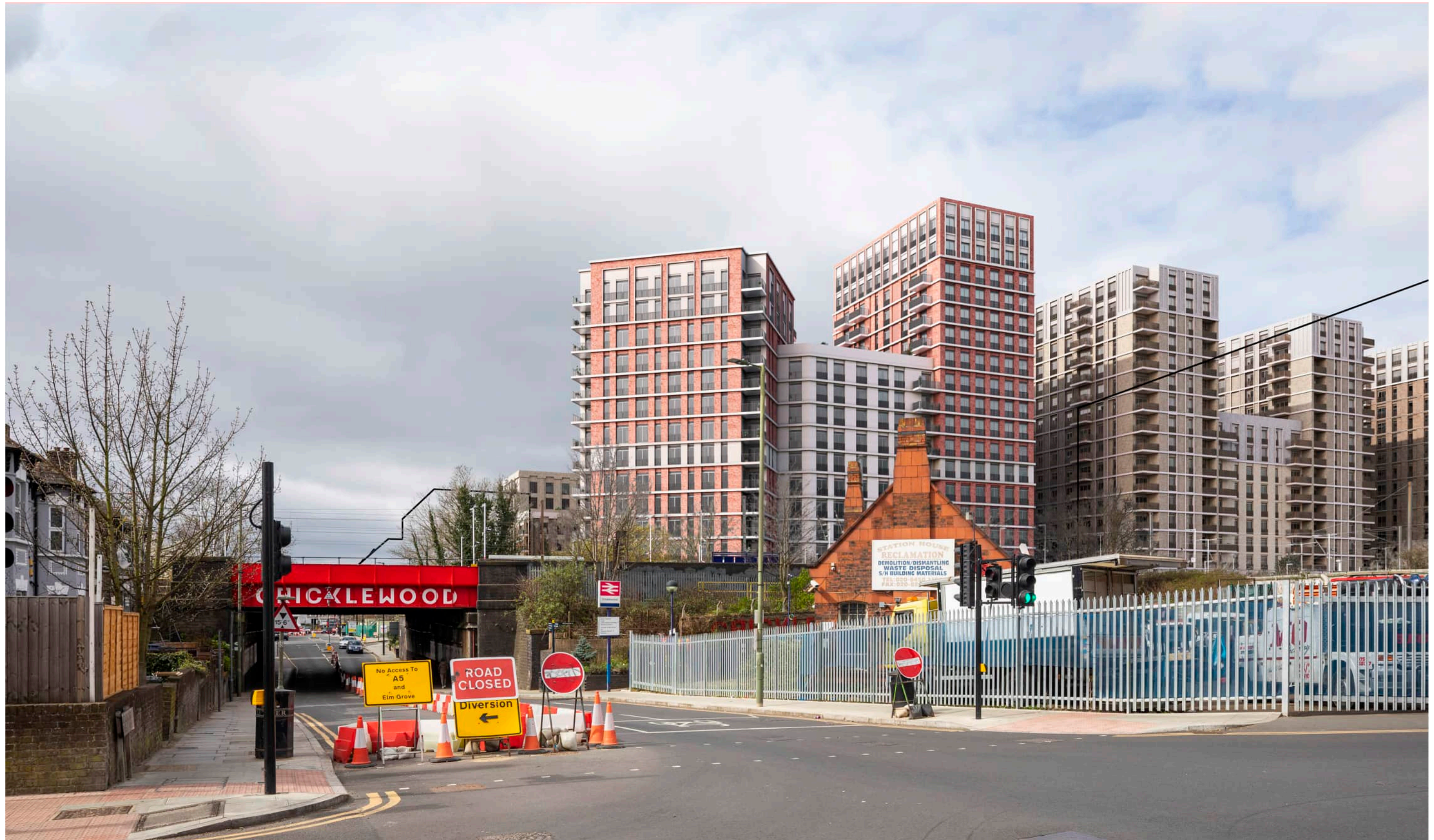
Figure 6.25 View 5 -Illustrative scheme towards Cricklewood Station looking south west - also showing the cumulative massing of 1-13 Cricklewood Lane, demonstrates that the Illustrative Application scheme is an elegant and legible addition to the town centre
