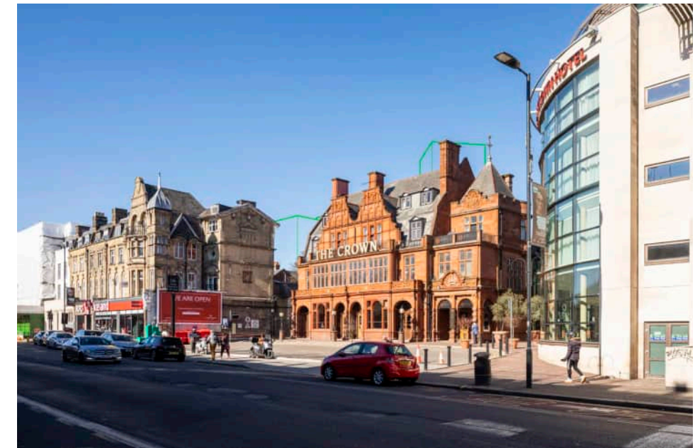
Figure 6.32 View 8 - The Crown Pub. Wireline view of the Original Scheme.
