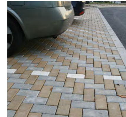
Figure 7.44: Permeable block paving
