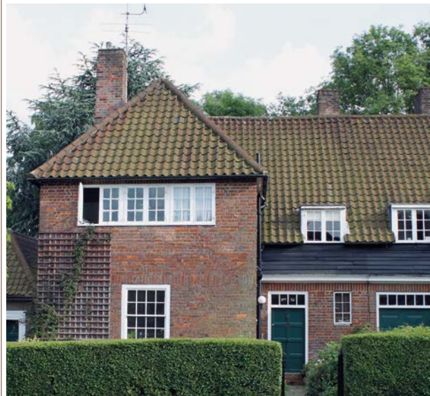
▲ A pantiled roof.
