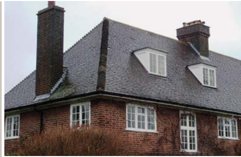
▲ New dormers that sit effortlessly on a substantial roof.
