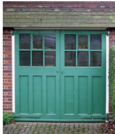
▲ An original timber garage door with glazed upper panels.
