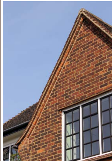
▲ Tile and brick detail at the verge of a gable.
