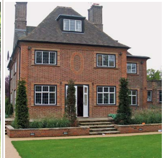
▲ A two storey extension carefully detailed to respect the host building.
