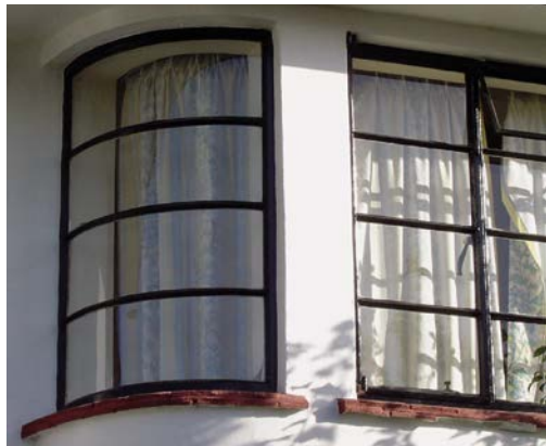
◀ Curved steel corner windows were common in the 1930s.
