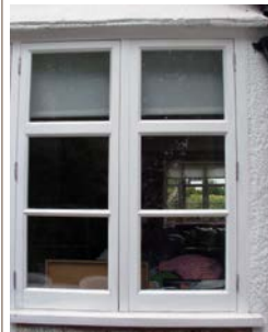
▲ A replacement timber window. This is double glazed but detailed carefully to accurately match the original.
