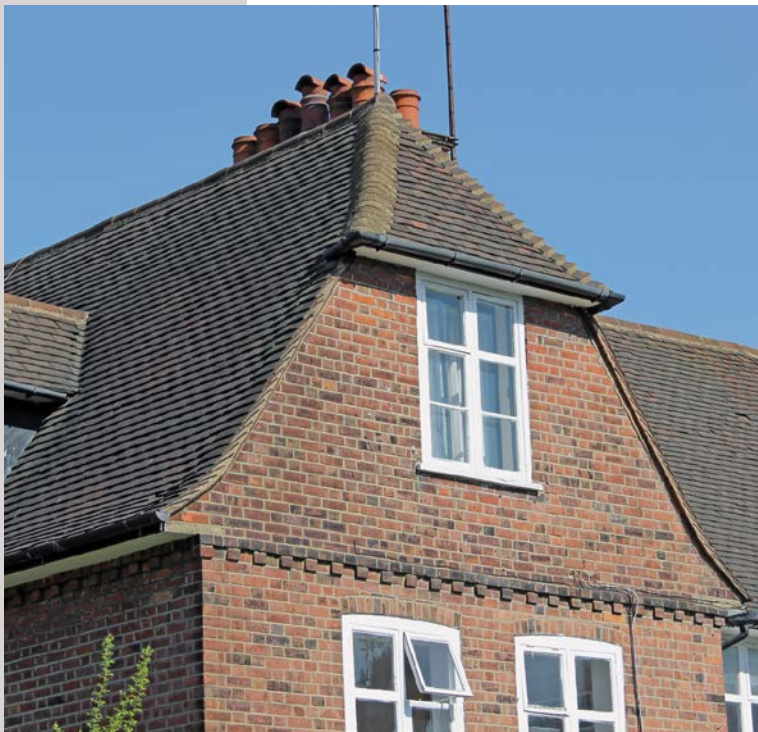
▲ A steeply sloped tiled roof is characteristic of Suburb houses.
