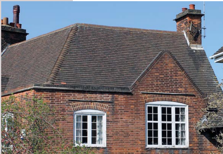
▲ Parapet and coped gable on Willifield Green.
