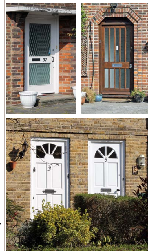
▲ These replacement front doors, in a range of standard styles, look very poor and are no substitute for the carefully designed originals.
