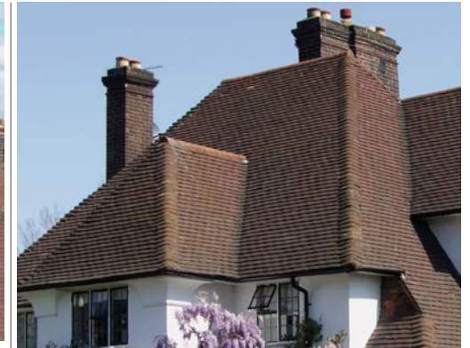
▲ Bold hipped roof with bonnet tiles.
