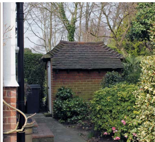
◀ Attractive brick sheds were often built to house garden tools.
