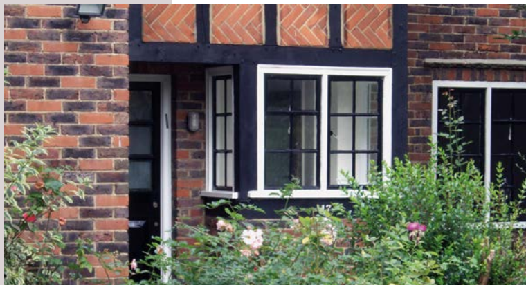
◀ Steel cottage windows.
