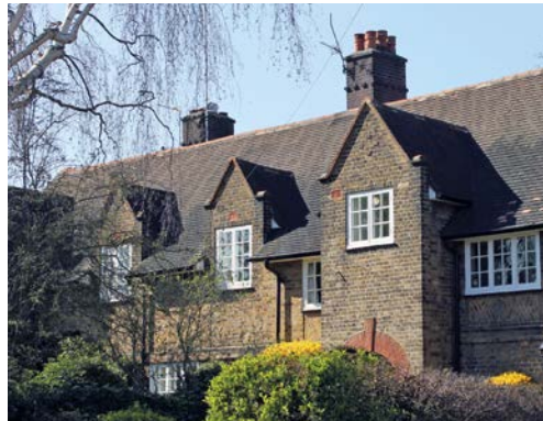
▲ Bold hipped roof with bonnet tiles.
