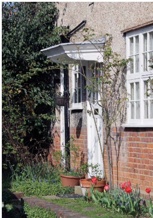
▲ Examples of flat roofed door canopies.
