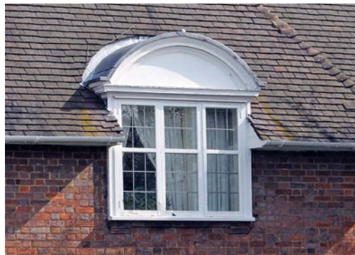
◀ Half dormer with segmental pediment.
