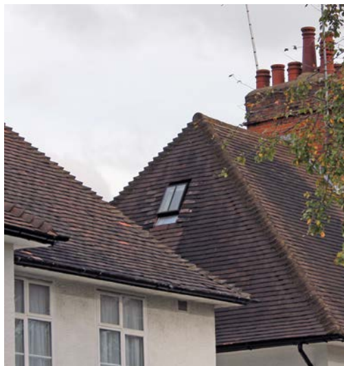
▲ A small conservation rooflight on a side roof slope.
