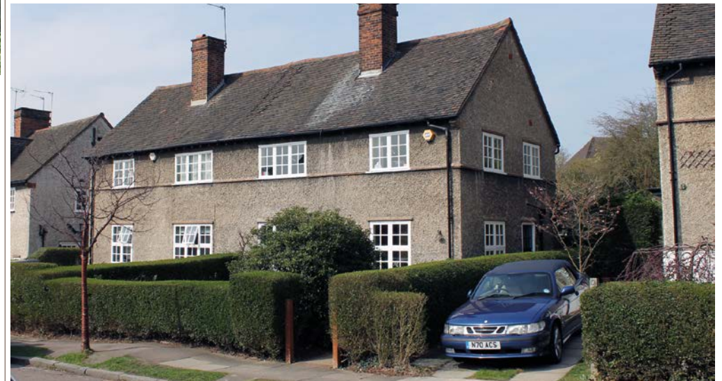
▲ The mellow appearance of unpainted roughcast.
